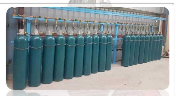
**Gas Manifold** is a group of Gas Cylinders connected in series and is designed to supply gas through a pipeline to an equipment or building.
